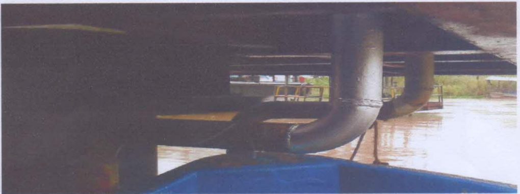
Picture showing facility after repair.
